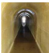
SprayWall is a self-priming polyurethane lining that reinstates structural integrity while providing infiltration control and chemical resistance. SprayWall's guick curing time allows the newly protected structure to be returned to service shortly after the application is completed,
