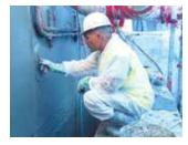
GeoCast™ Geopolymer Mortar is a microsilica geopolymer with fly-ash binder, pozzolan powder, polymermodified and fib-r reinforced mixture with select admixtures for rehabilitation of horizontal concrete pipes, corrugated steel culverts, sewer manholes, and water treatment plant structures. The chemical resistant GeoCast™ withstands hydrogen sulfide corrosion and offers special additives for marine environments.
