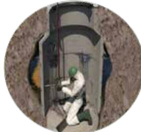
Prime Flex 920 is a single-component polyurethane injection resin used to seal gushing leaks, including wide gaps, in concrete where the structure isn't subject to movement. This hydrophobic, super-low-viscosity polyurethane reacts with water and expands to form a closed cell, watertight, rigid foam. Also used for permeation grouting.
