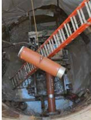
NO-DIG jacking pipe from Logan Clay Products is preferred for Pilot Tube Method of Guided Boring installations. Vitrified clay jacking pipe provides unsurpassed axial strength of 18,000 psi and greater. VCP-J eliminates the need for a casing pipe that remains in the ground. See a sample in booth #707.
