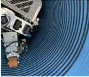
Manufactured In-Place Composite Pipe (MICP) is an innovative trenchless pipeline rehabilitation system that robotically builds a new structural pipe within the host pipe. NSF 61 approved and up to 250 Psi, MICP offers a cost-competitive solution to rehabilitate large-diameter pipelines with minimal public disruption and minimal loss in system performance.
