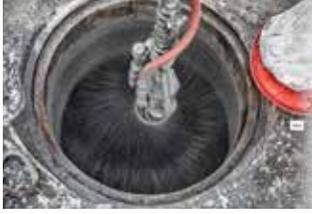
The Mainstay Composite Liner is a rehabilitation system consisting of a high-strength restoration mortar and an epoxy corrosion barrier coating that are applied and cure simultaneously to repair and protect underground infrastructure. The mortar and topcoat become tightly bonded not only to the substrate, but also to each other.
