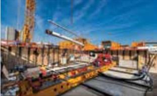
E-Power Pipe® is used for the trenchless installation of small-diameter product pipes at shallow depths. Over long distances of up to two kilometers, both pressure-resistant and non-pressure-resistant product pipes are installed quickly, safely and precisely. The two-stage process integrates aspects of the proven horizontal directional drilling (HDD) technology and pipe jacking (microtunnelling).
