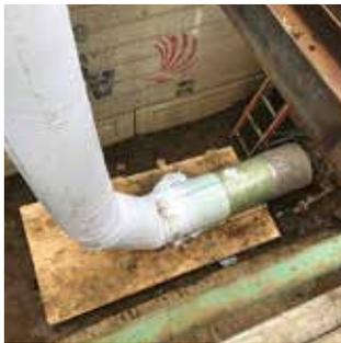
Aegion continues to advance the pipeline rehabilitation market by offering the latest innovations in cured-in-place pipe (CIPP) technology specifically engineered for drinking water applications. The InsituMain™ System, our showcase CIPP innovation for pressure pipe renewal, is a composite material of polyester fiber, fiberglass, and a specially formulated epoxy resin system.
