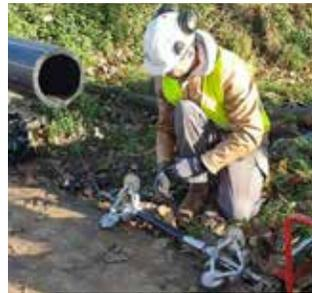
Take no risk; get it mapped! Reduct gyroscopic mapping tools are passed through your pipe/duct, resulting in a 3D XYZ as-built map that can be immediately uploaded into any GIS-platform, as well as highly accurate bend radius and inclination measurements.
