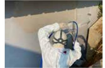
Hydroplate 6500 is the premier epoxy lining for concrete and steel in aggressive wastewater environments. Its ultra-durable, high-build design and single-leg application provide outstanding longevity, low permeability, and superior chemical resistance. It achieved excellent ASTM G210 results, complies with AWWA C210, and offers a return to service of 10 hours.
