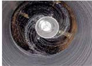
Spray-in-place-pipe is an emerging technology that uses high-pressure spraying of durable material (cement mortar, polyurea, or epoxy) to coat the inside of a pipe using a spray head controlled by a computerized spray rig. Warren Environmental will have a spin head and a coated pipe on display during UIC.
