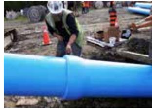
For HDD and static pipe bursting projects, get the job done efficiently with AquaSpring™ C900 Certa-Lok® RJIB pipe. It's designed for trenchless applications with robust tensile strength for pulling multiple segments underground. AquaSpring™ C900 Certa-Lok® RJIB pipe is now available in sizes up to 18".
